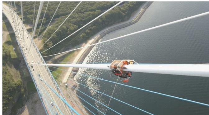
**Figure 9** Intros MH 120-300 at the stay-cable of the bridge in Vladivostok (Far East)
